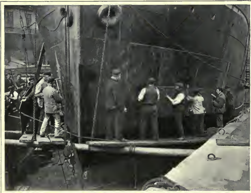
RIVETTERS AT WORK (UNION DOCK, LIMEHOUSE).
