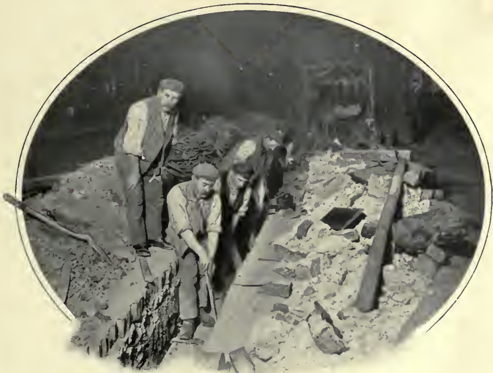
NIGHT WORKERS LAYING AN ELECTRIC CABLE.
